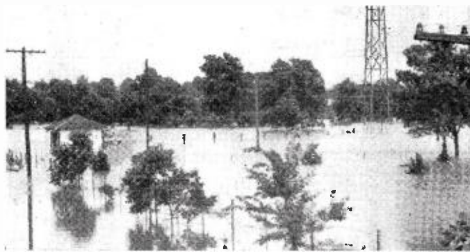
WATER EVERYWHERE , the most in 15 years, inundated the transmitter site of KHBC, Okmulgee, Okla., throwing the station off the air 45 hours. Water was 2½-feet deep in the transmitter house at left and the tuning house was completely submerged.
